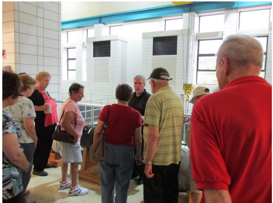
McGhee describing the different types of pipes the Commission uses in the pipeline system
